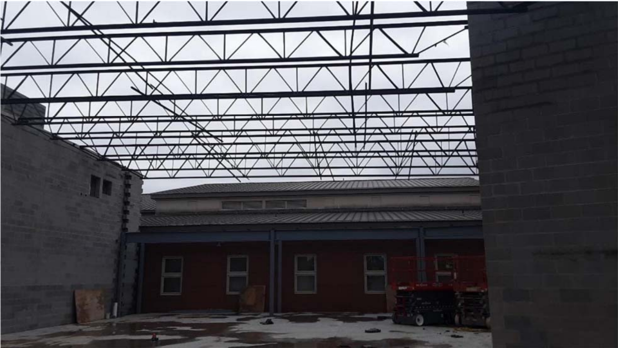
North & East Gym walls
